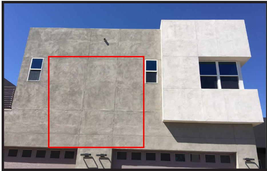
Horizontal and/or vertical stucco control joints
