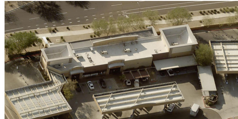
*Image from County in Peoria, Arizona of reverse oriented pumps.
