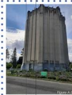
The Lincoln Heights Reservoir Tank #1
