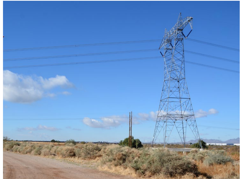
EXISTING OVERHEAD UTILITY LINES
