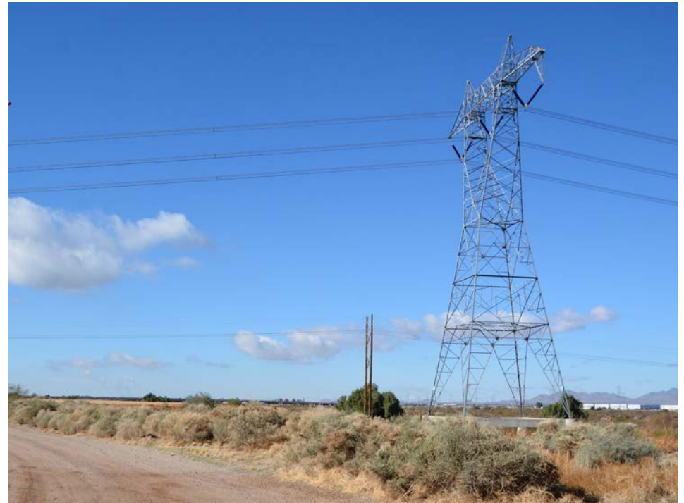
EXISTING OVERHEAD UTILITY LINES
