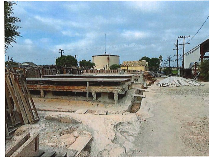
Concrete Paver production area and "runoff" (Photo taken by J. Munoz on September 12, 2024)
