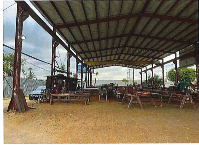
Steel Fabrication area "Large Parcel" (Photo taken by J. Munoz on September 12, 2024)
