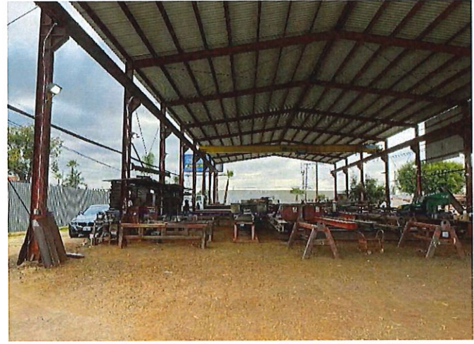
Steel Fabrication area "Large Parcel" (Photo taken by J. Munoz on September 12, 2024)
