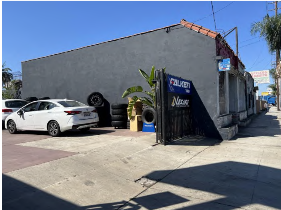
Photograph 3. Overview of east elevation, facing southwest.
