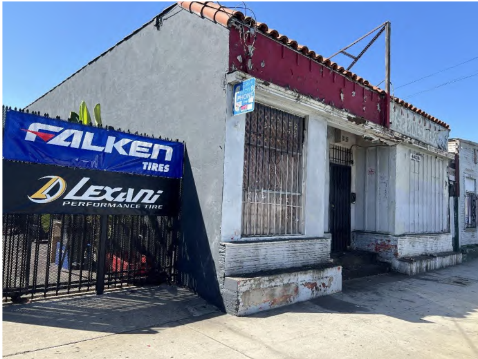
Exhibit 5. Overview of Building 1, view southwest
