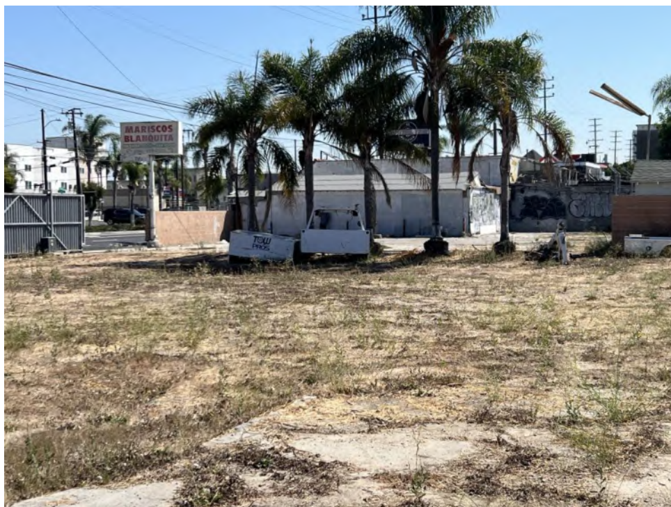
Photograph 5. Overview of parking area and field adjacent to subject property, as well as metal entry gate and freestanding sign, facing northeast.
