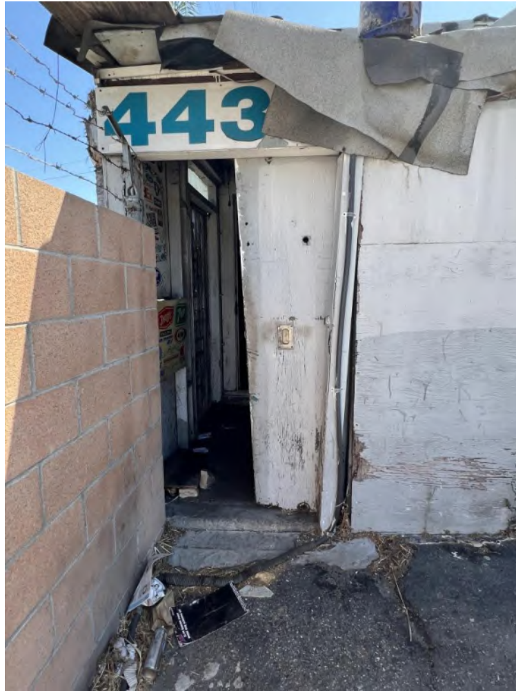
Photograph 3. Detailed view of entryway on west elevation, facing east.
