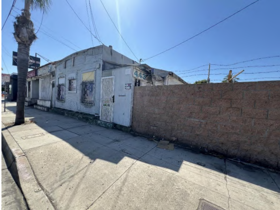
Exhibit 4. Overview of buildings within project site, view east
