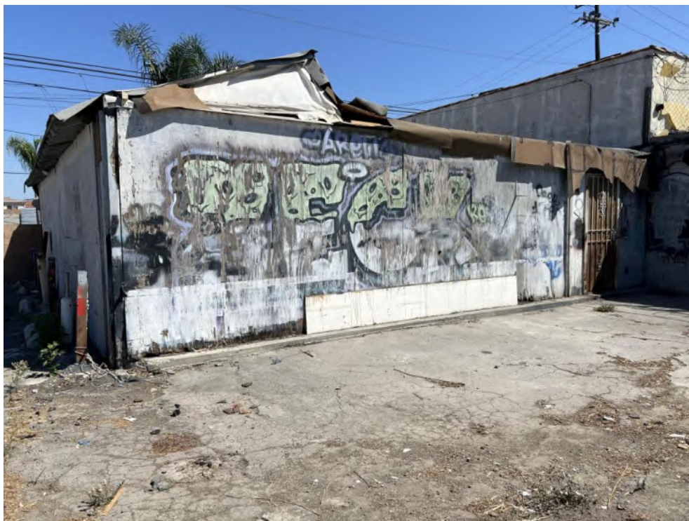
Photograph 4. Overview of south elevation, facing northeast.
