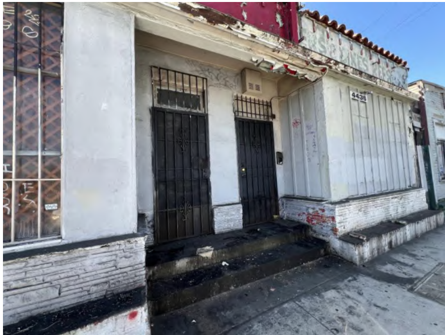
Photograph 2. Detailed view of entry doors on primary elevation, facing southwest.
