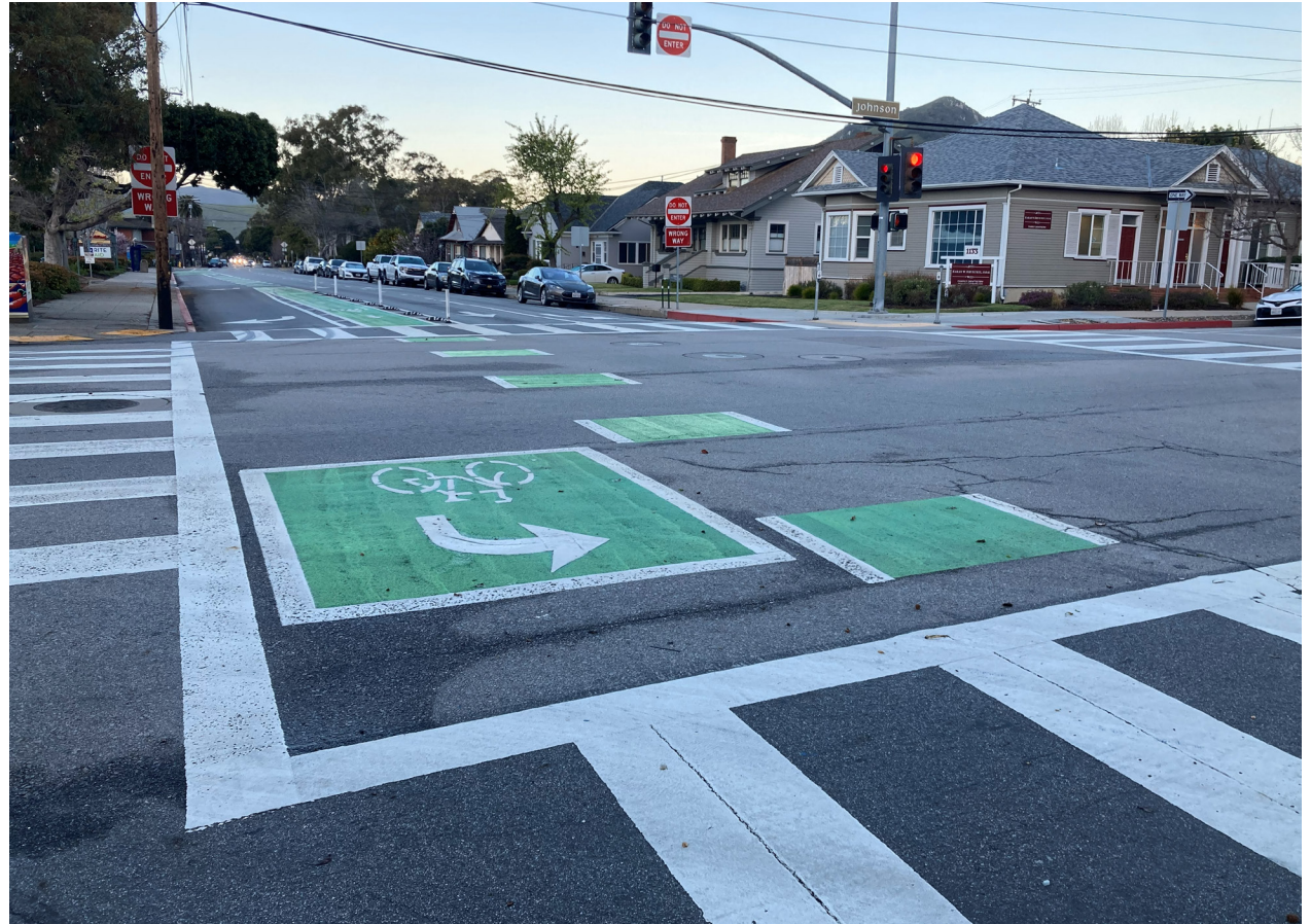
Exhibit 88. Example of a bicycle box in San Luis Obispo, CA
