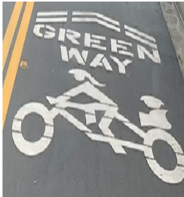
Exhibit 90. “Greenway” shared lane marking on a bike boulevard in San Luis Obispo, CA
