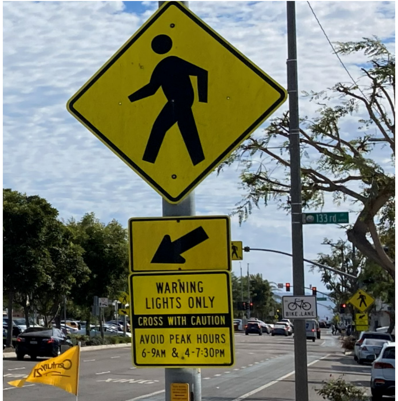
Exhibit 91. Non-MUTCD-compliant crosswalk signage on Hawthorne Blvd
