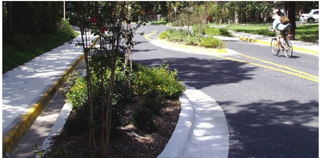
Exhibit 74. Permanent chicane with median island (source: Los Angeles Department of Transportation)
