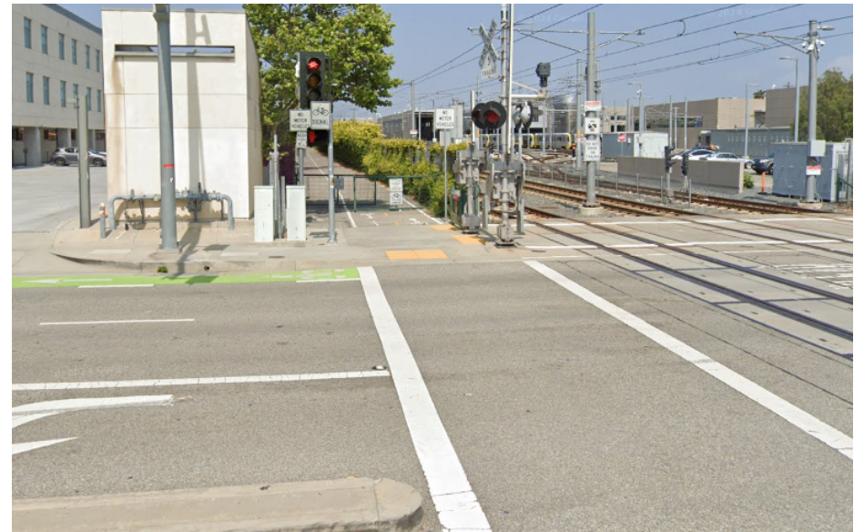
Exhibit 17. Example of an existing Class I shared-use path crossing (Santa Monica, CA)
