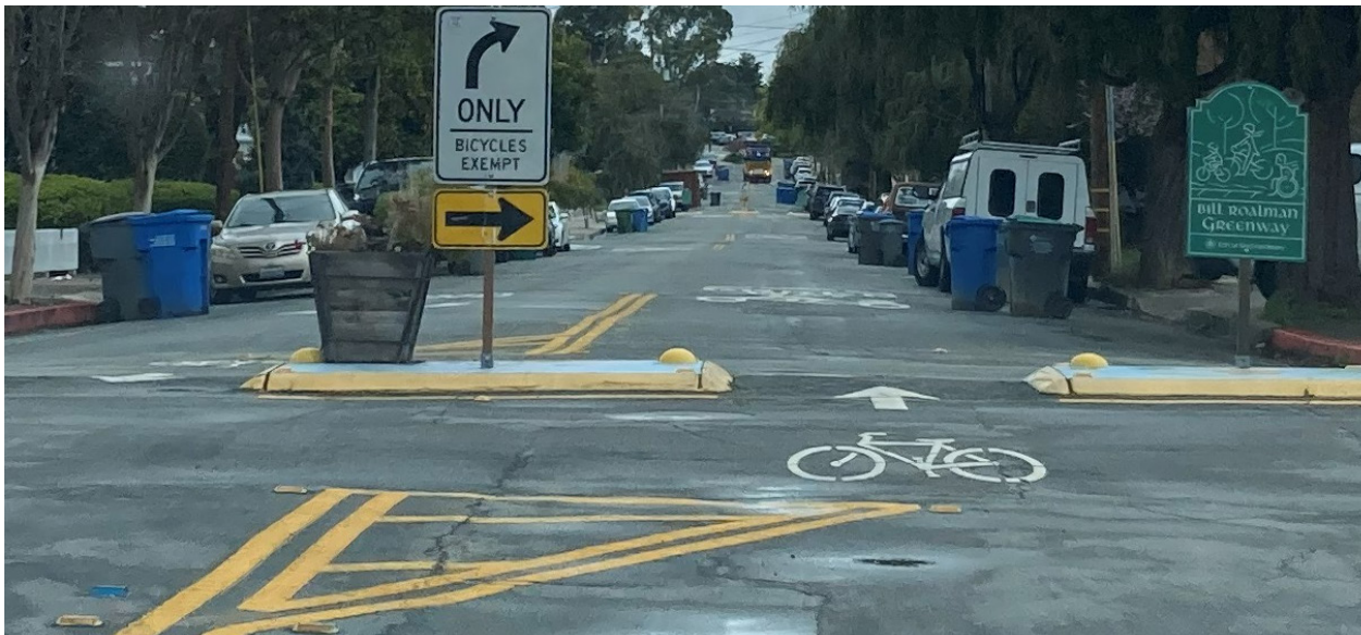
Exhibit 7. Existing Class III bike boulevard in San Luis Obispo, CA (source: GTS)
