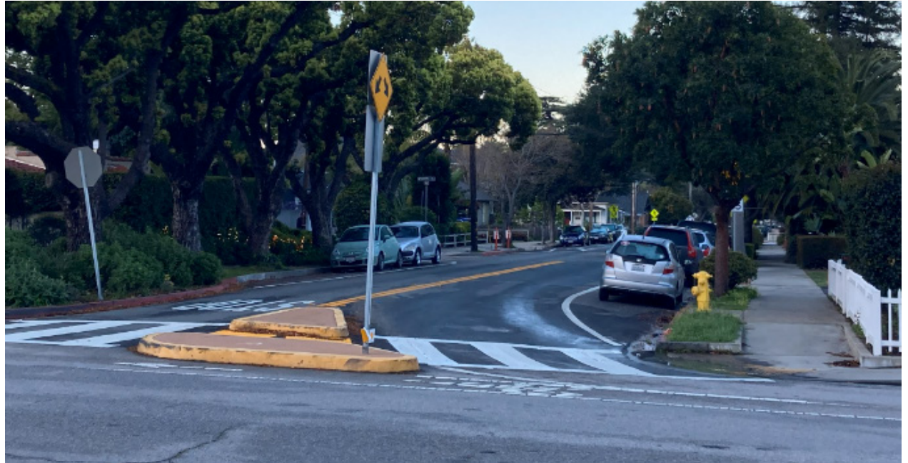
Exhibit 83. Permanent forced turn island preventing left turns from a major road to a residential street in San Luis Obispo, CA
