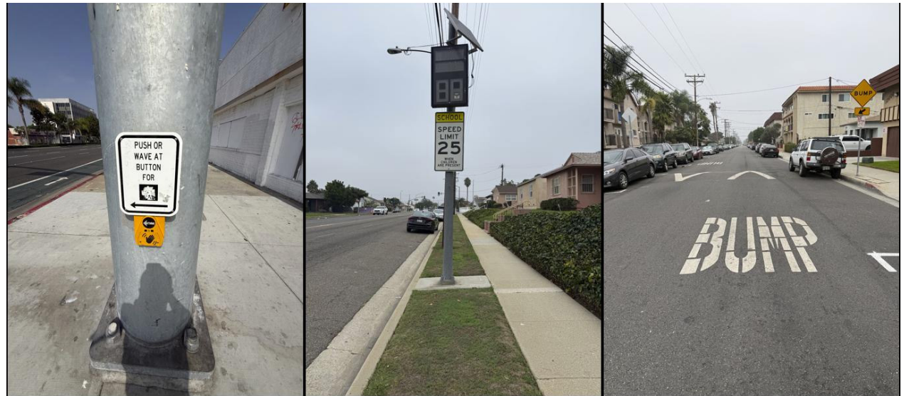
Exhibit 11. Safety devices in Hawthorne: accessible pedestrian signal (left); dynamic radar sign (center); speed hump (right)
