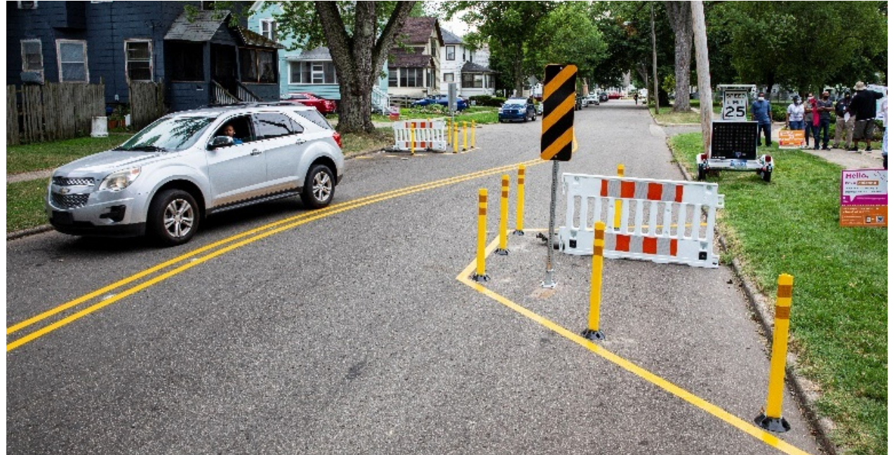
Exhibit 73. Temporary chicane (source: MLive)
