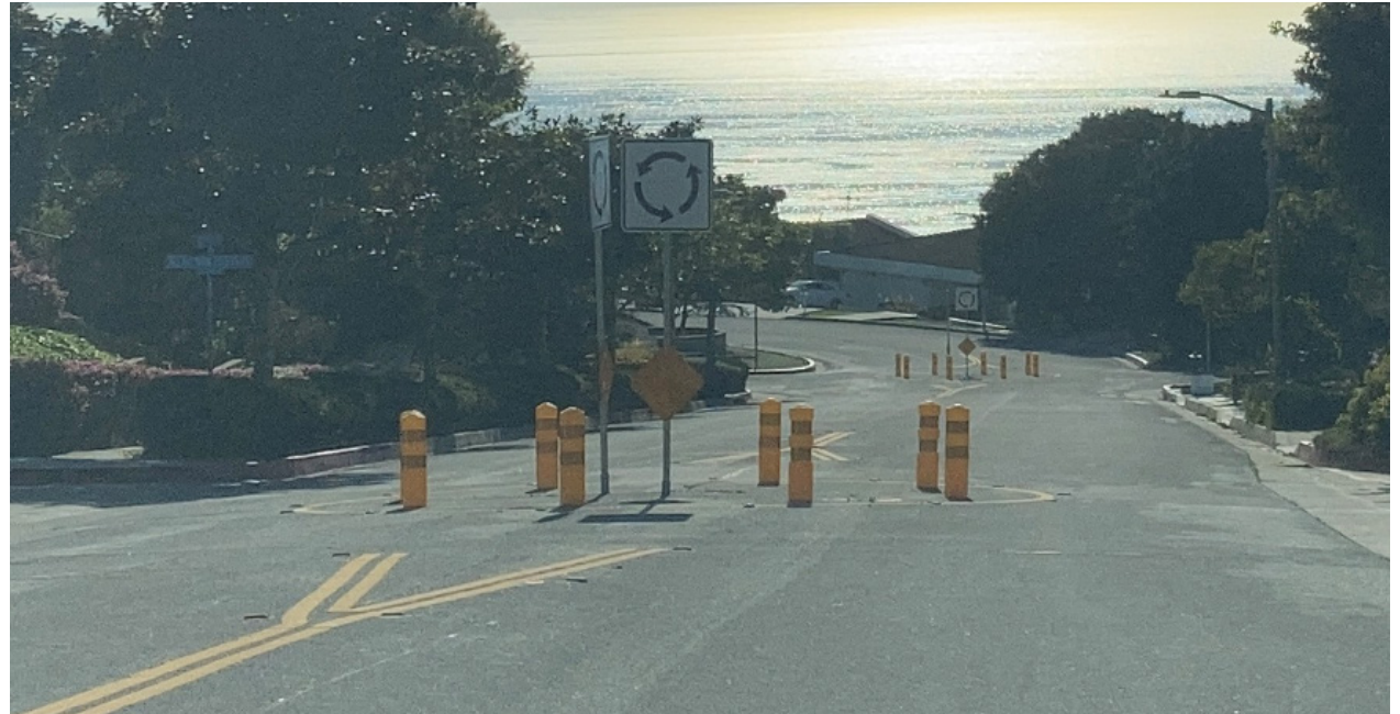
Exhibit 75. Temporary traffic circle in Rancho Palos Verdes, CA
