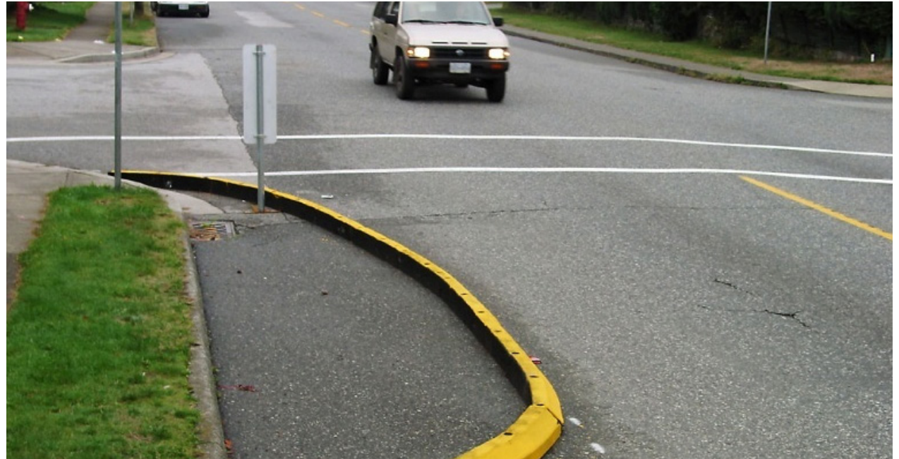
Exhibit 69. Temporary curb extension (source: Wikimedia)
