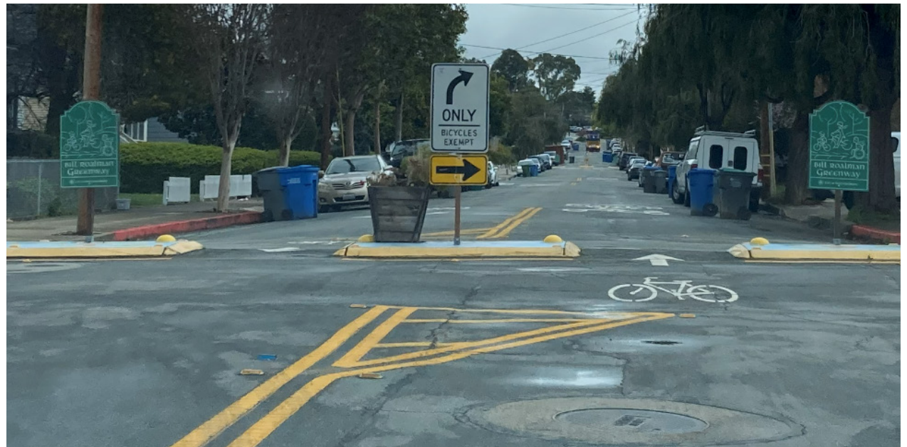
Exhibit 82. Permanent modal filter with mountable curbs, preserving emergency access in San Luis Obispo, CA
