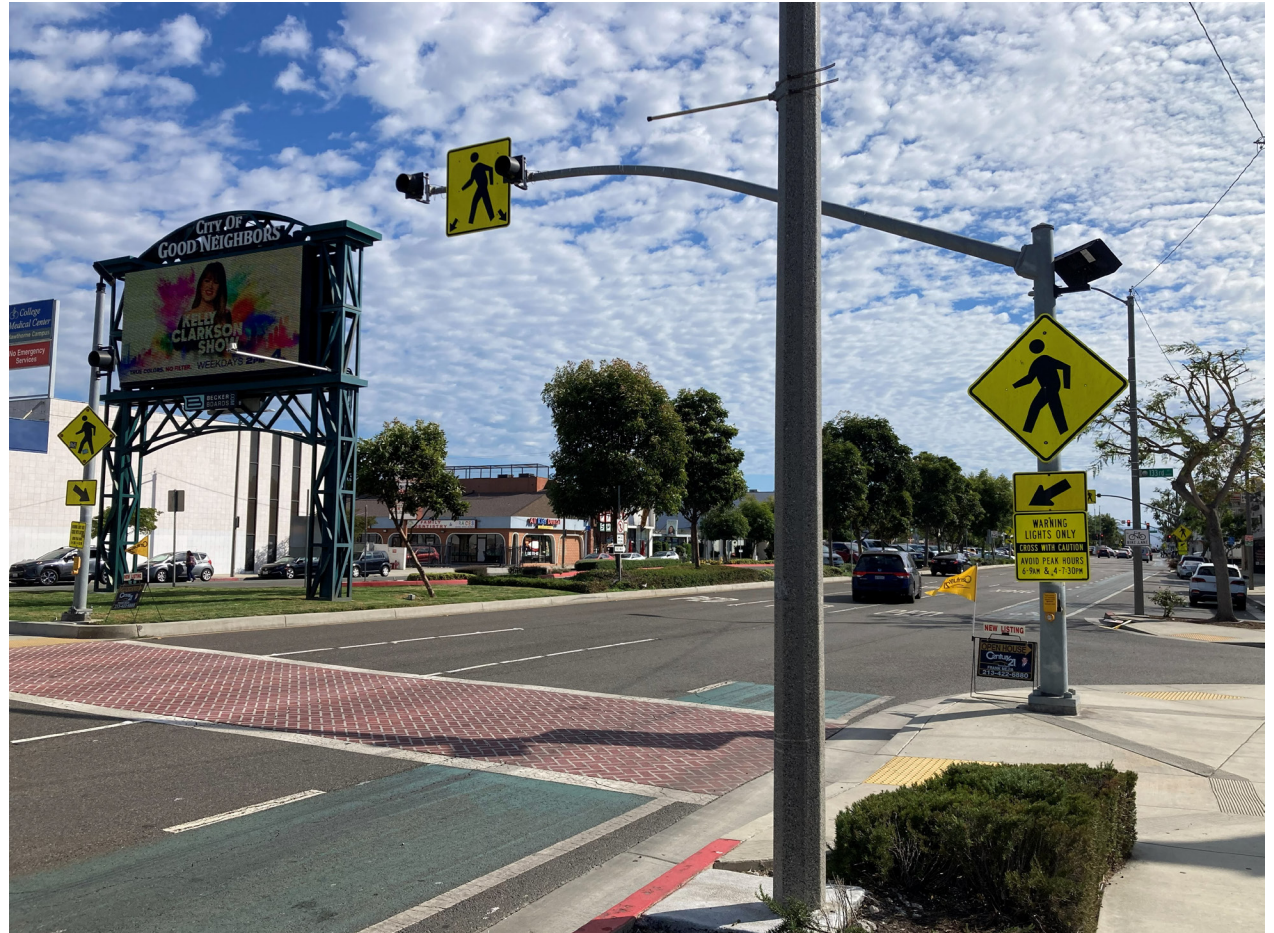
Exhibit 10. Mid-block crossing on Hawthorne Blvd with “peak hour” signage
