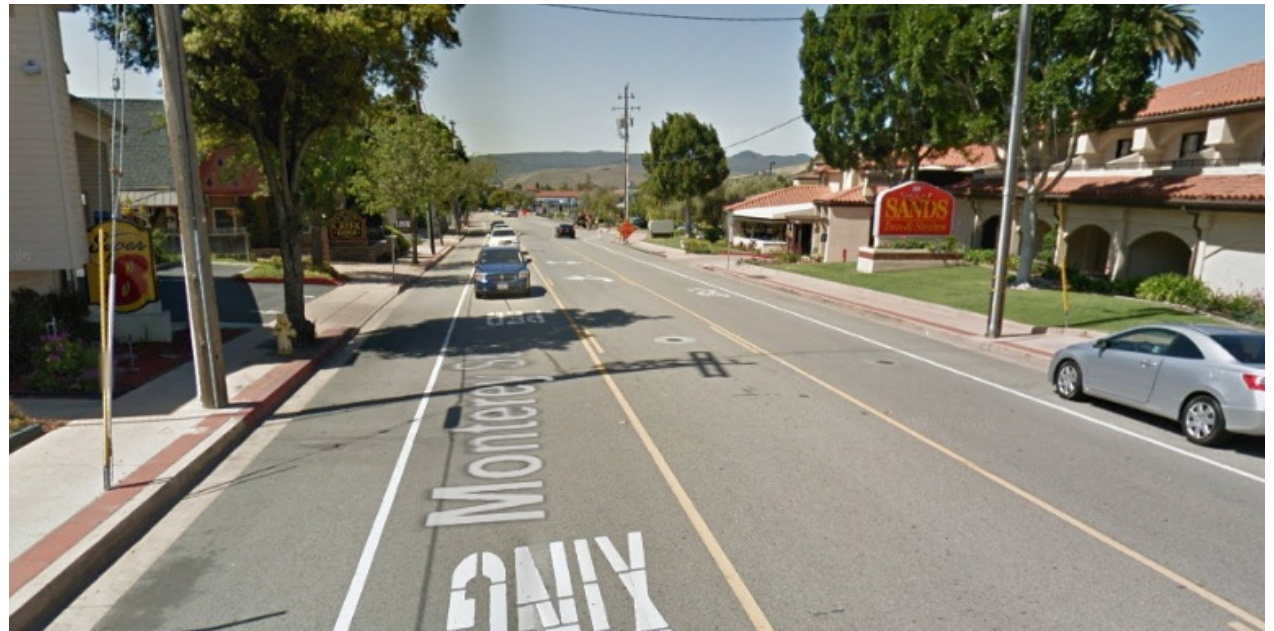
Exhibit 85. Before (above) and after (below) views of a street where lane restriping created optical narrowing (source: Google Street View)
