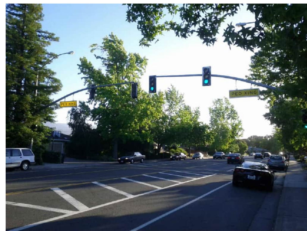
1 Mid-Block Pedestrian Signal
