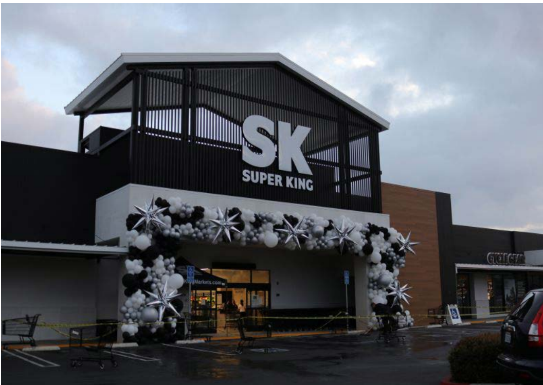
Before and After - Big Box Retail stores often have sufficient economic utility to be repurposed for other retailers rather than be converted to housing. This example from Culver City on Sepulveda Boulevard shows a Big Lots store converted to Super King Markets in April 2026.
