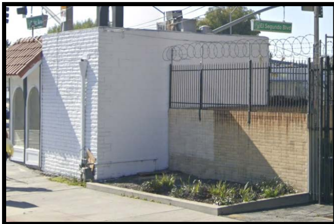
View of existing north building wall (looking southwest)
