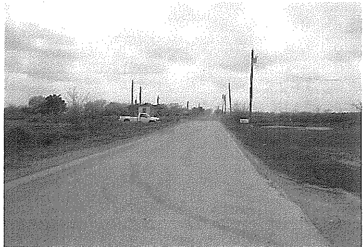
Photo 6 Southern view of Mile 2 West.
