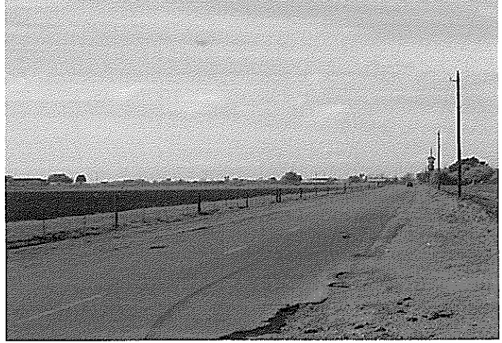
Photo 6 Southern view of Mile 2 West.
