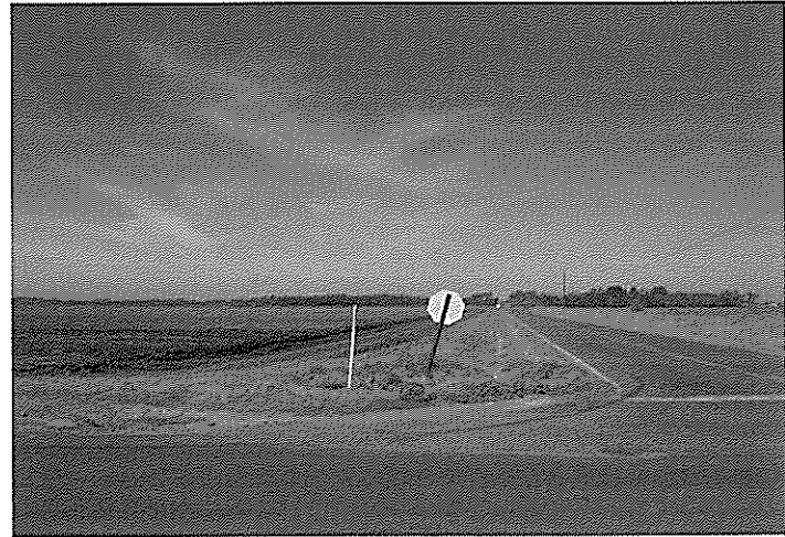
Photo 8 Western view of the NWC of Mile 8 and Mile 2 Roads.
