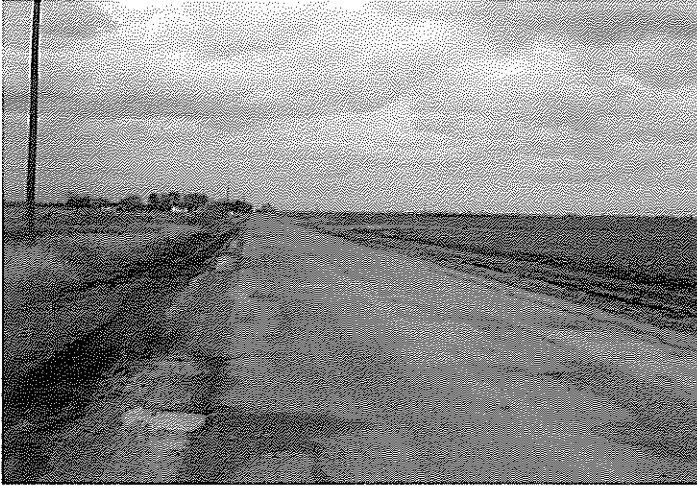
Photo 5 Northern view of Mile 2 West.
