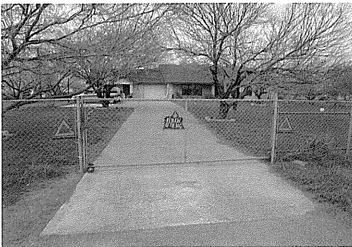
Photo 7 Western view of concrete drive and sliding chain link gate located within the part to be acquired.
