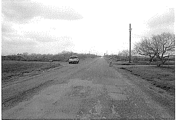
Photo 6 Southern view of Mile 2 West.
