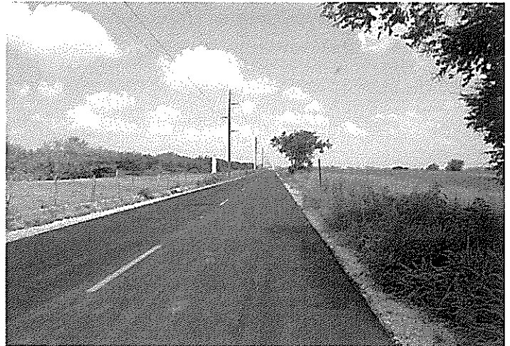
Photo 6 Western view of Mile 17 1/2 North Road.
