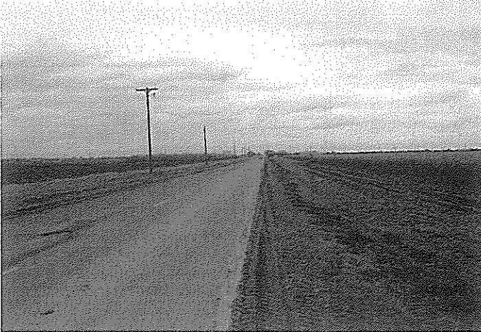
Photo 5 Northern view of Mile 2 West.
