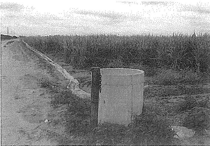
Photo 7 Eastern view of stem pipe with irrigation system located within the part to be acquired.
