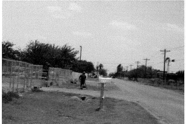
Photo 4 Southern view of Cesar Chavez Road.
