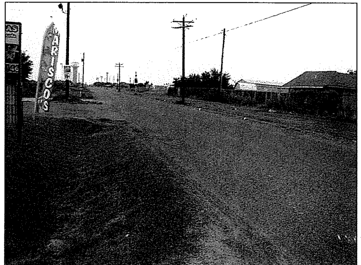
Photo 4 Western view of Eldora Road along the frontage of the subject property.
