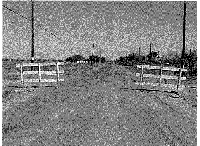
Photo 4 Northern view of Tower Road
