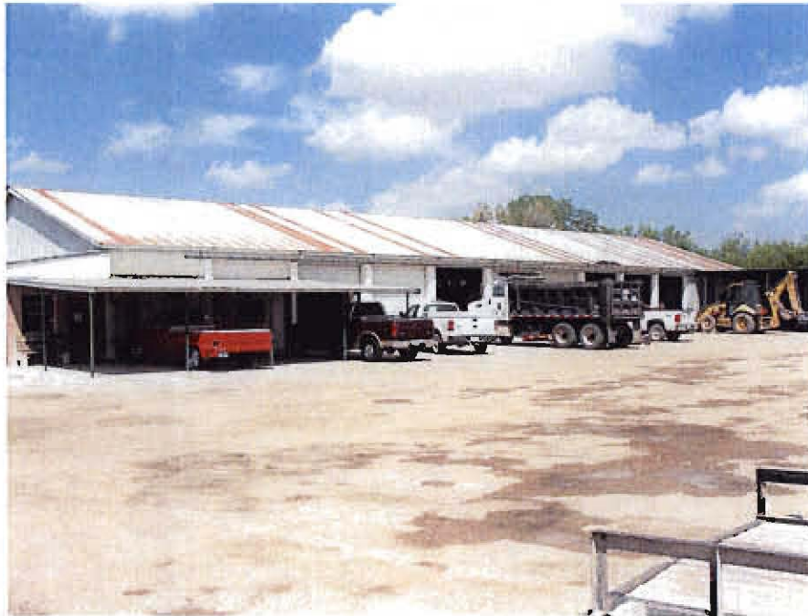
Western view of the main building structure.
