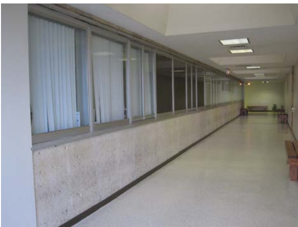
Original exterior ribbon windows remain on the second and third floors, enclosed in the corridors of the 1980 addition.
