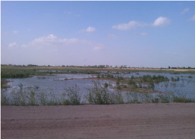
Photo 3 View of detention pond in use.
