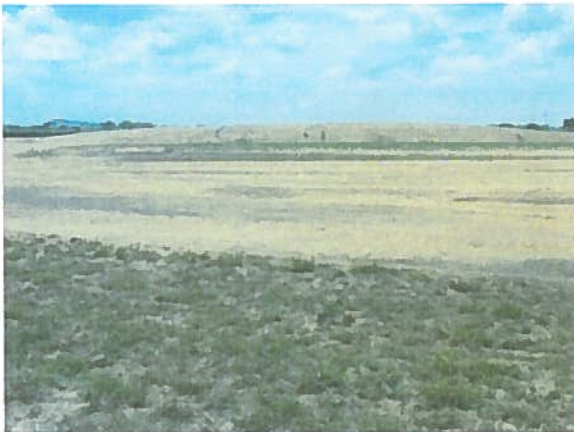
Clearing of project site, stockpiling of dirt in background.
