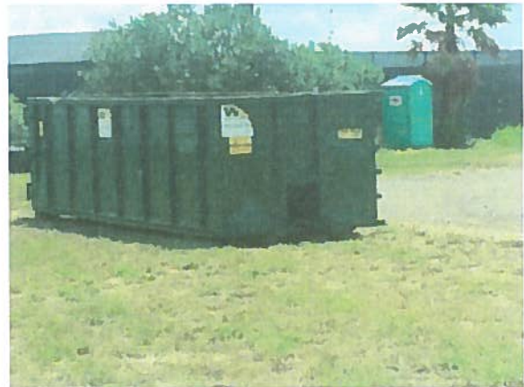
Trash dumpster and port-a-potty delivered to job-site.
