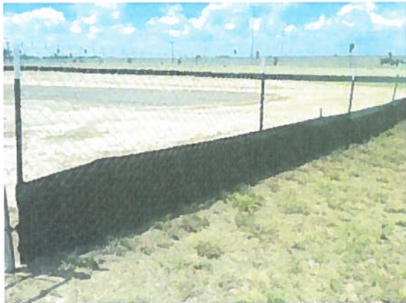
Erosion control/chain link fencing placed along site perimeter.
