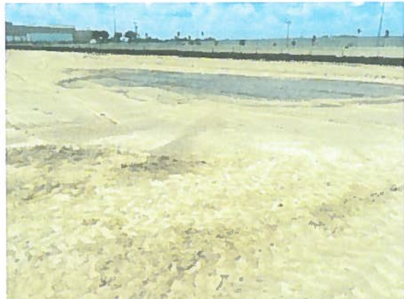
Earth work and grading of detention pond at west perimeter.
