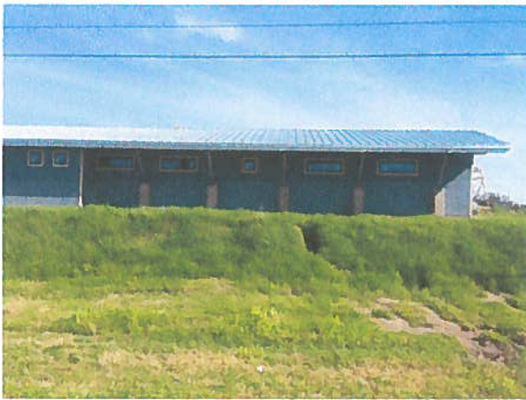
South elevation as see from Highway 107.
