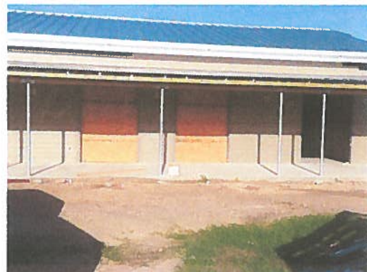
Courtyard view of multi-purpose room and porch area.
