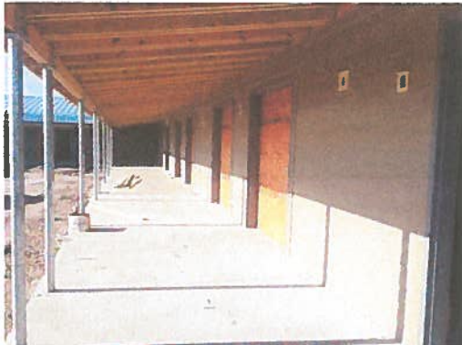
Porch at Multi-purpose Room, roof and decking in-place.
