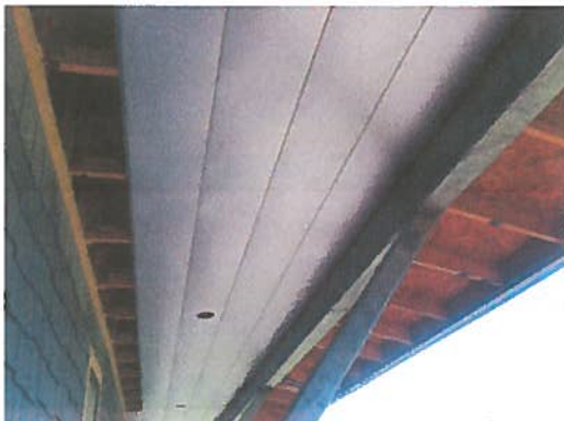
Metal soffit installation continues along south elevation.
