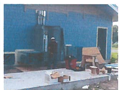
Electrical and HVAC tie-ins.
