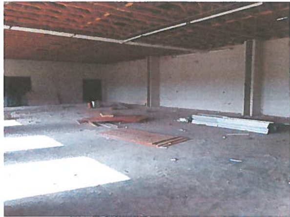
Gypsum drywall installation begun in all areas, multi-purpose room – above.
