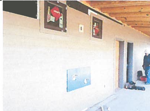
Windows and Hardie-panel sidings installation completed.
