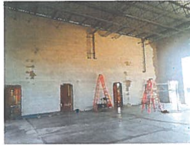
Interior walls of apparatus bays.
