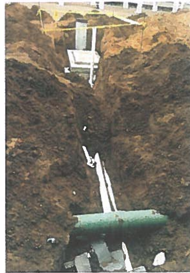
Plumbing line installation, south side.
