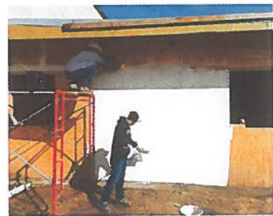
Air barrier applied to plywood exterior.
