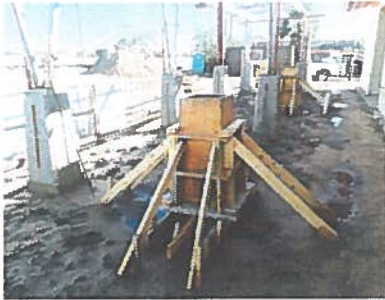
Concrete chapes, reformed, repoured.
