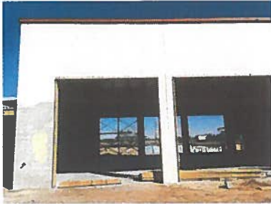
South wall of apparatus bay.
