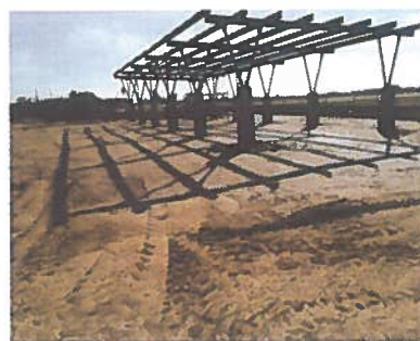
Truck port, priming of structural members.
