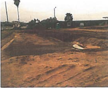
Detention pond site work in place.
