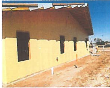
Air Barrier installation on east wall.
