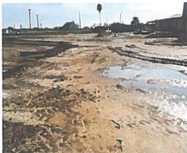
Shaping of north detention pond.
