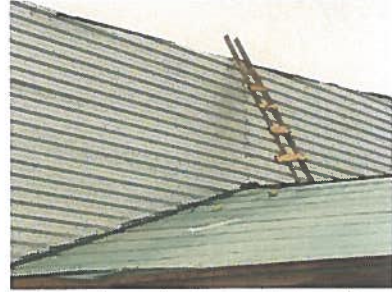
Metal wall panels along roof slope/ridge.
