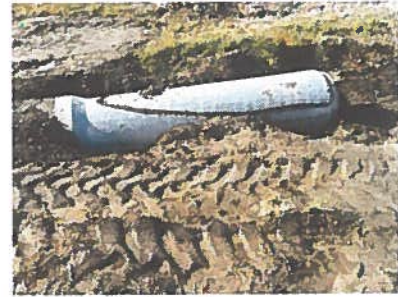
Concrete pipe installation, detention pond.
