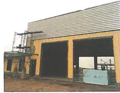
Metal wall panels at apparatus bays.
