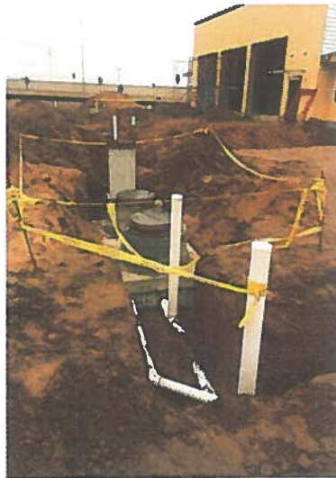
Grease trap installation, south side.
