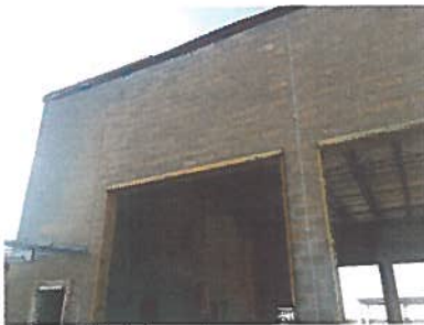
Concrete block walls at apparatus bays.
