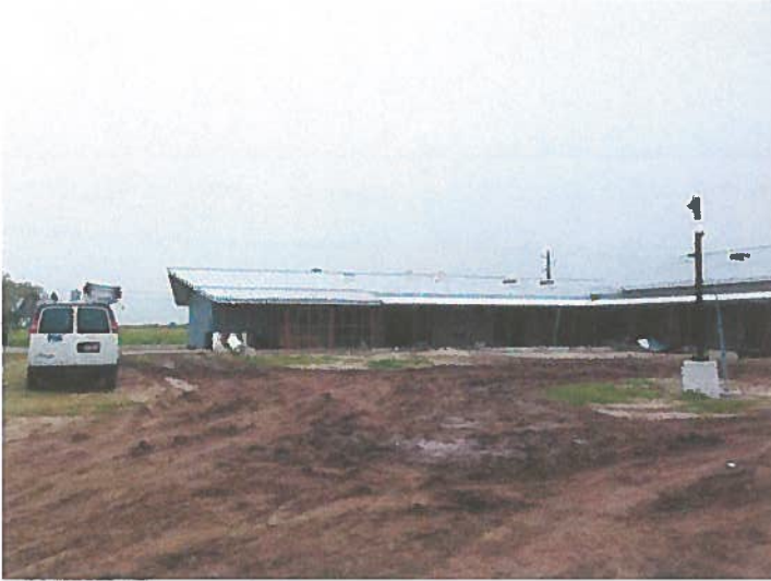
Current condition of site
