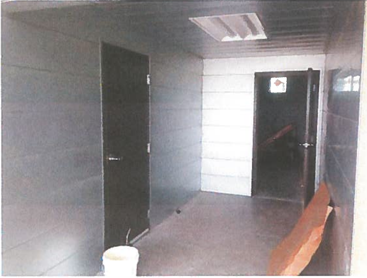
Hall 108 finished metal cladding
