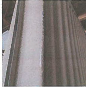
Installed folding partition. Partition slat is damaged.
