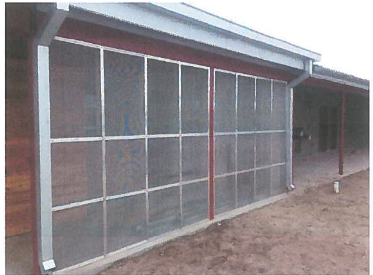
overall mesh screen / oversize downspouts
