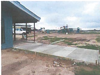
Poured sidewalk at entry.
