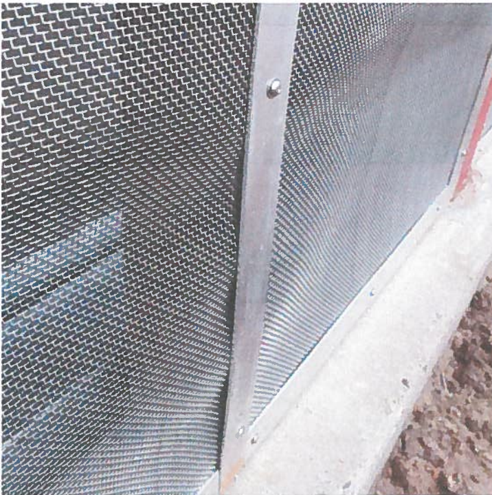
Bad install leaves creases in plan of mesh
