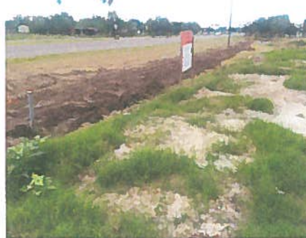
Utility-line installation by North Alamo Corp.
