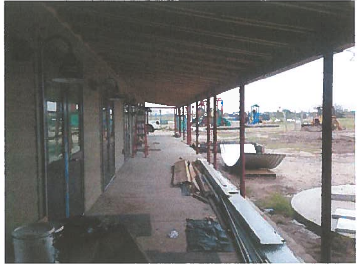
view down corridor
