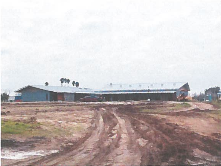
Current condition of site
