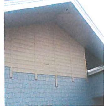
Metal soffit installed at eaves.
