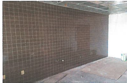
Ceramic tile wall at multi-purpose kitchen.
