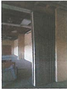
Installed folding partition. Partition slat is damaged.
