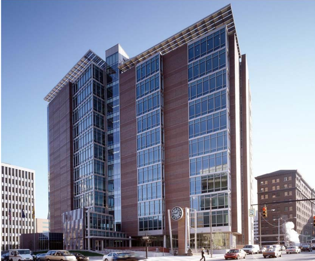
Kent County Courthouse, Grand Rapids, Michigan
