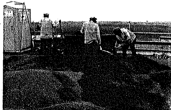
The collected gravel was shoveled into a bucket for removal from the roof.
