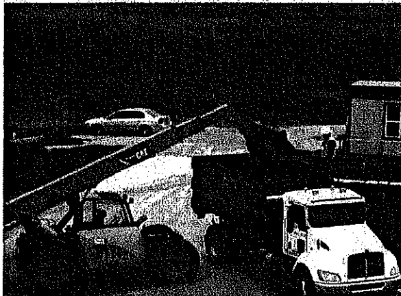
The buckets of gravel were emptied into the back of a dump truck and hauled to the storage location.
