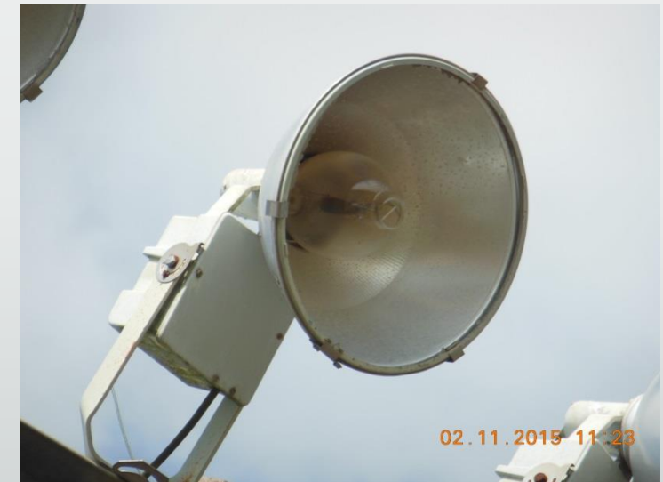
Exterior lights susceptible to vandals and weather
