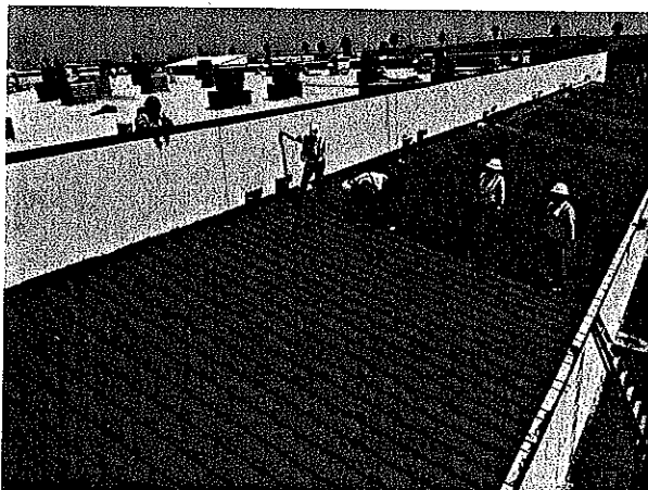
Tinsmiths were in the process of installing the new metal roofing at the front of the facility.
