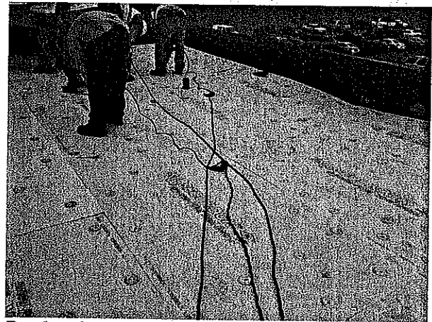
Roofers installed a layer of 4'x8'x½" gypsum fiber roof board over the entry roof.
