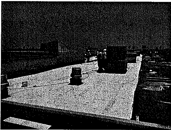
Roofers continued installing the new cover board and base ply onto the roof labeled Fox.
