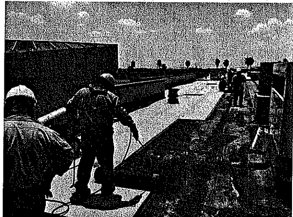
*Roofers began installing POWERply® APP FR in the field of the roof labeled Fox.
