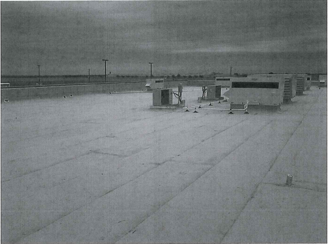
Final cap of roof placed at LEF
