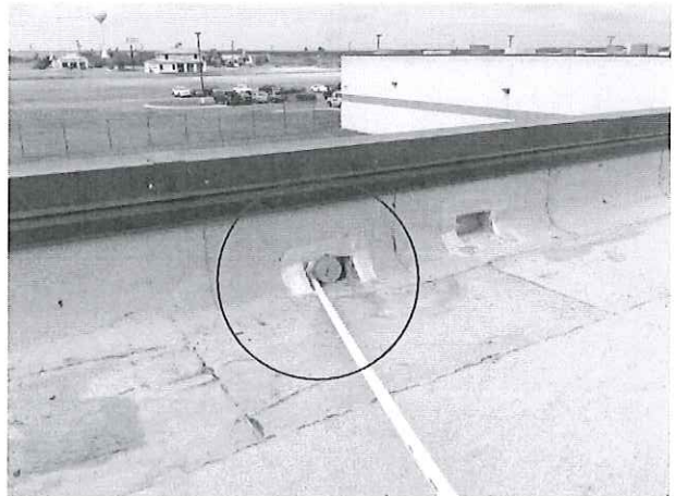
Ensure scuppers are clear of debris. Ensure condensation lines do not enter scuppers.
