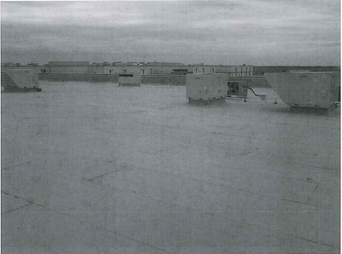
Final cap of roof placed at LEF
