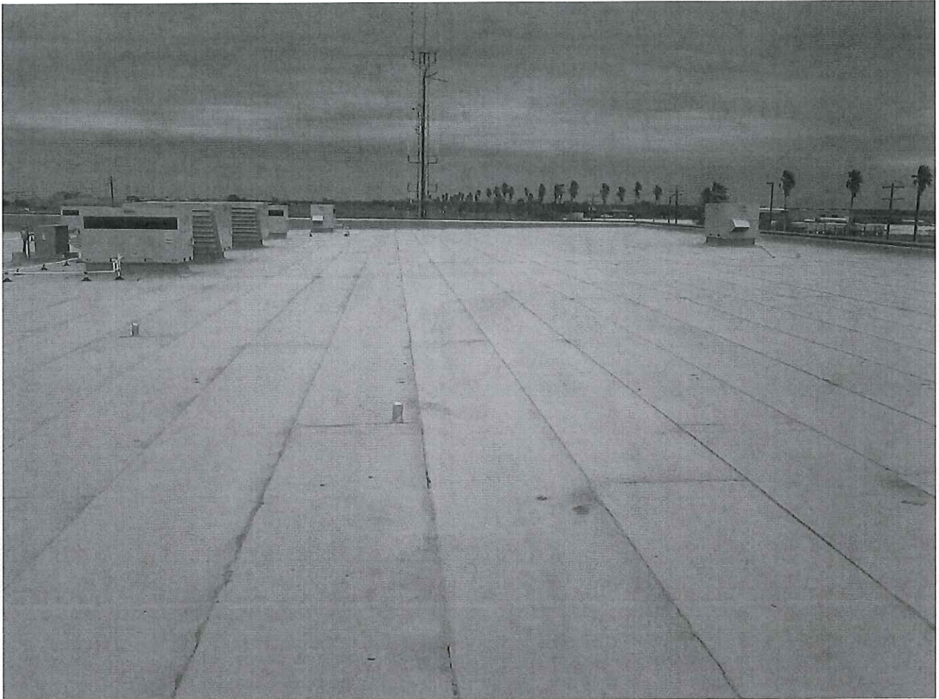
Final cap of roof placed at LEF
