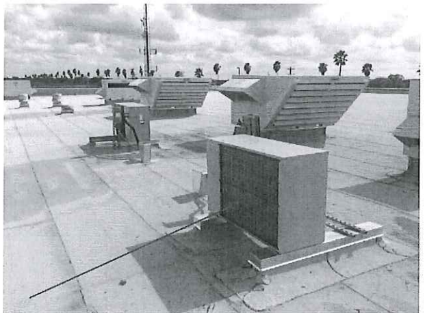
Secure the mini splits to the curbs on the LEC.
