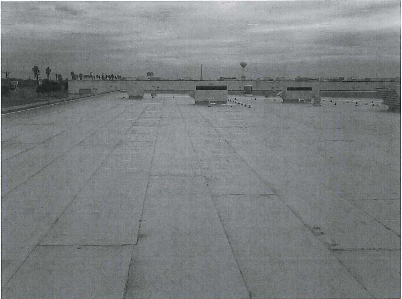
Final cap of roof placed at LEF
