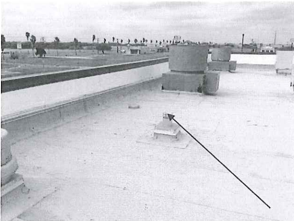
Install vent caps onto vents in the Alpha roof area.
