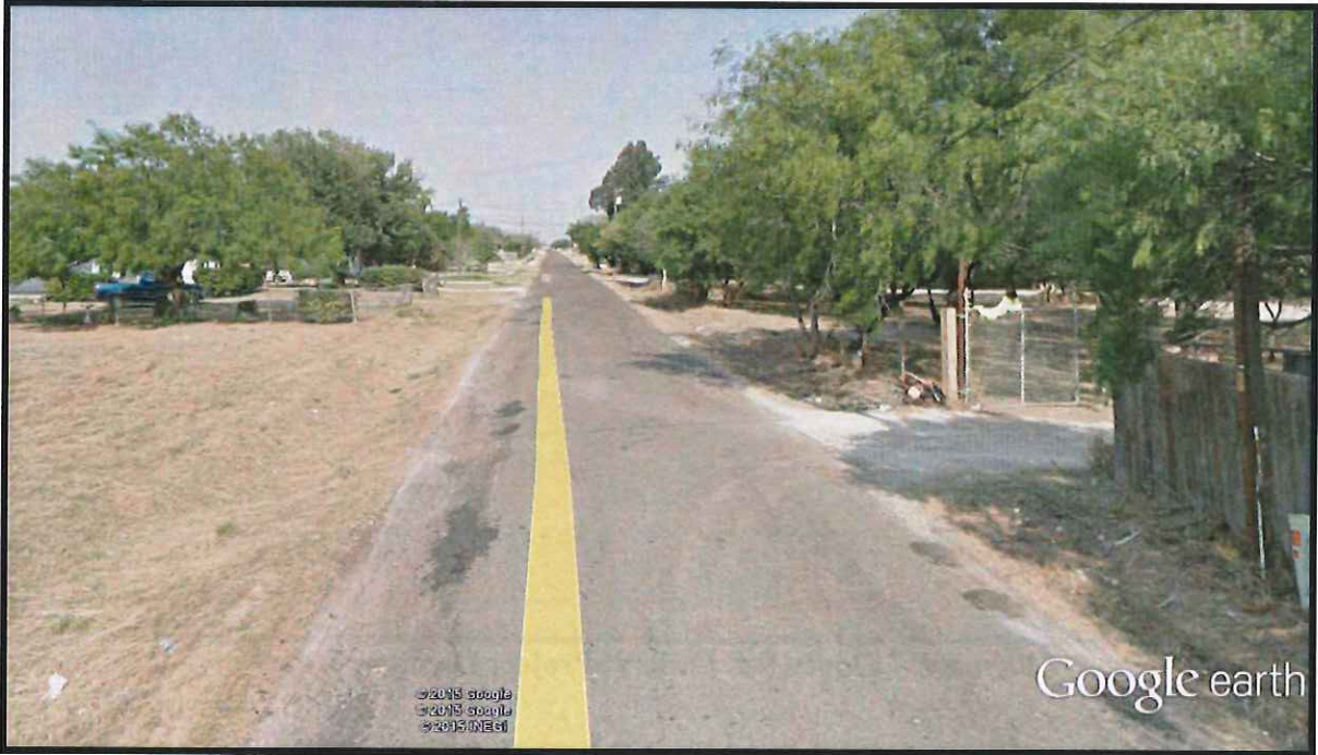
Figure 2B – Eldora Rd. Project Existing Corridor Photo
