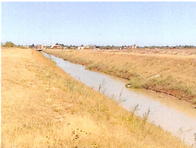
Photo 3 View of canal running through subject property.
