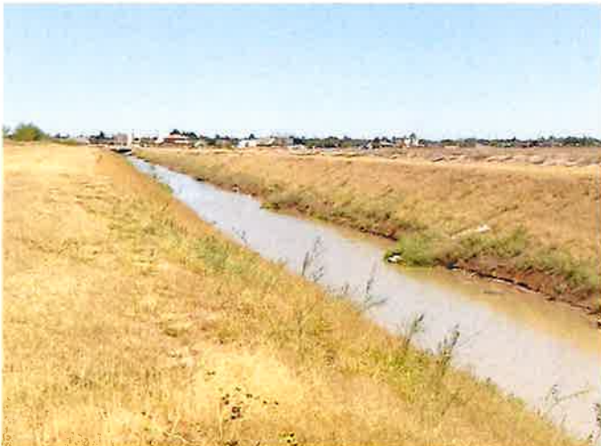
Photo 3 View of canal running through subject property.
