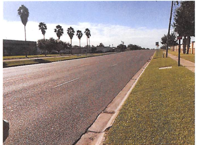
Photo 4 Southern view of Jackson Road.
