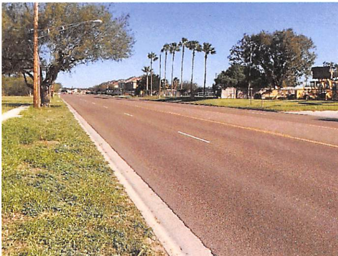
Photo 3 Northern view of Jackson Road.
