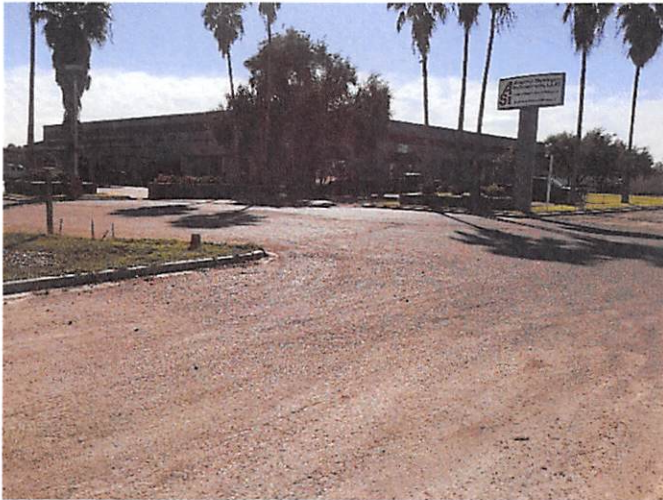
Photo 1 View of the subject property.
