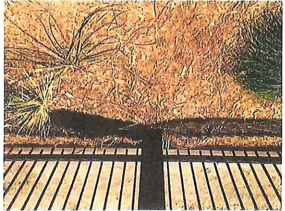
Plants were trampled during the installation of the perimeter wrought iron fencing by county crews. Landscaper will maintain, but not replace, during the next 30 days.
