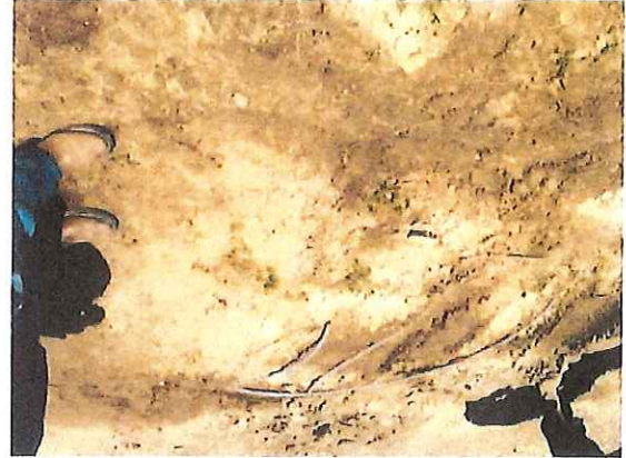
Irrigation drip-lines have been left exposed by county crews during the excavation of plumbing lines due to problems w/ sewage backing-up / unconnected lines of the CRC project.
