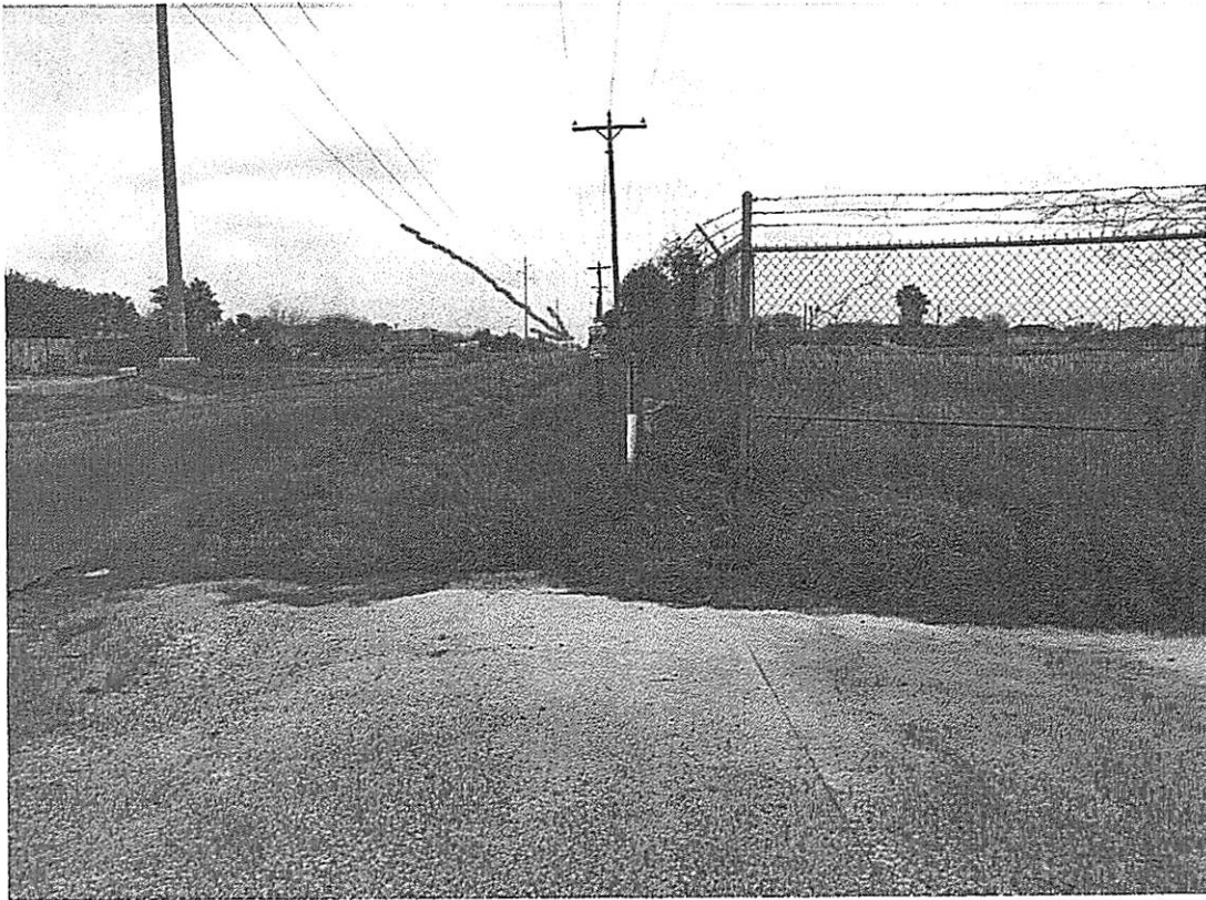
Under Ground Gas Line on the Westside of the Subject Property
