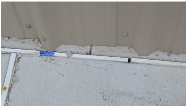
4.5 Caulk cracks and perforations.
