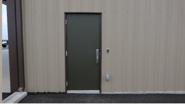
4.10 provide and install exterior signage.
