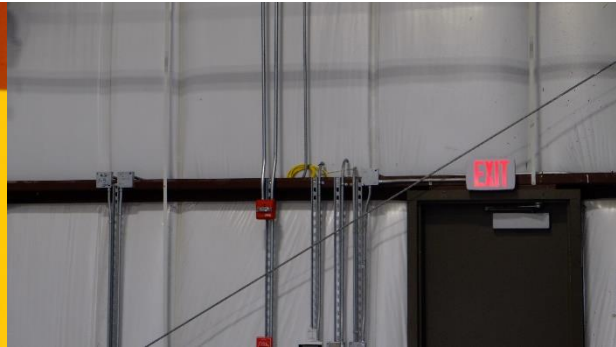
4.12 provide special systems conduit.
