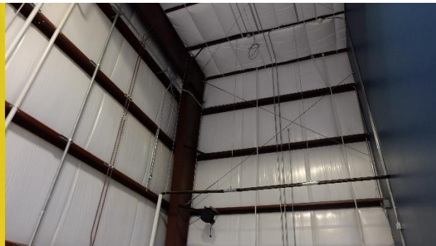
4.14 Provide and install to bay lights at tank area.
