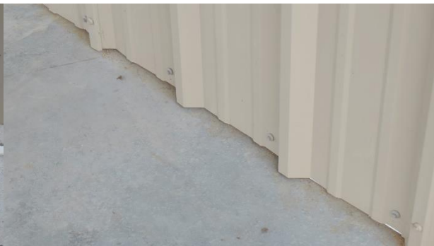
4.6 Caulk around perimeter to prevent water infiltration.
