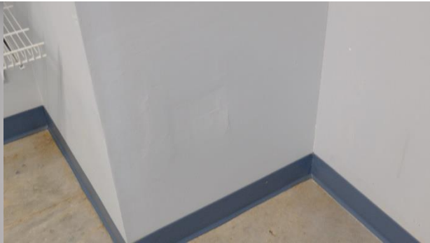
4.20 Smooth finish walls where needed. Apply 2 nd coat of paint throughout.
