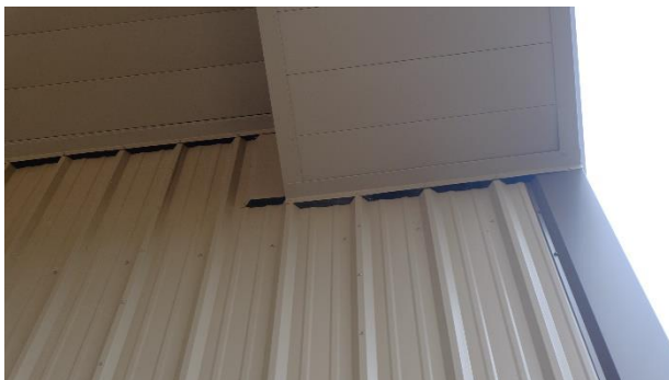
4.7 provide and install outside closures where missing.
