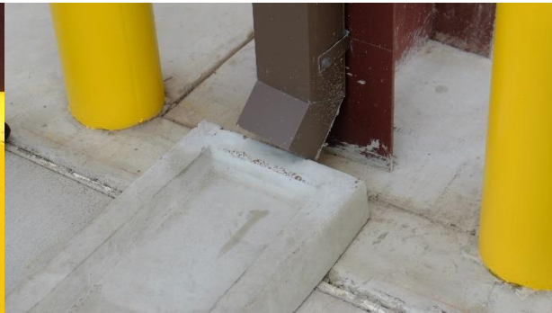
4.4 Adjust downspouts so the discharge to splash blocks.
