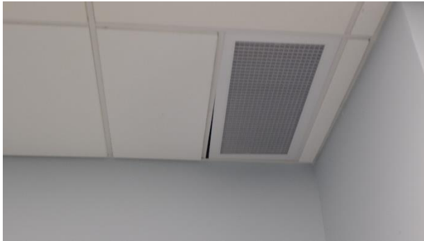
4.19 Adjust grid so no openings are visible.
