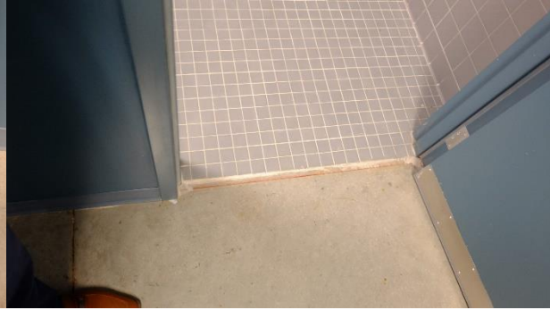
4.28 Provide and install transition threshold on shower room.
