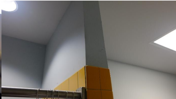
4.36 apply grout to uneven surfaces.
