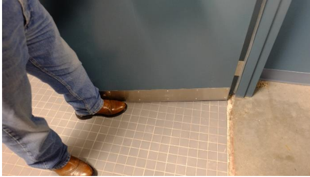
4.27 Provide and install transition threshold on restroom.
