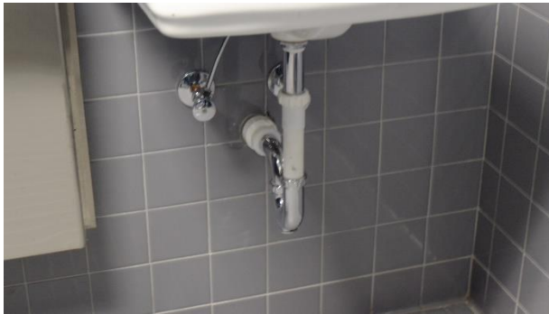
4.21 Install pipe insulation on restroom sink.
