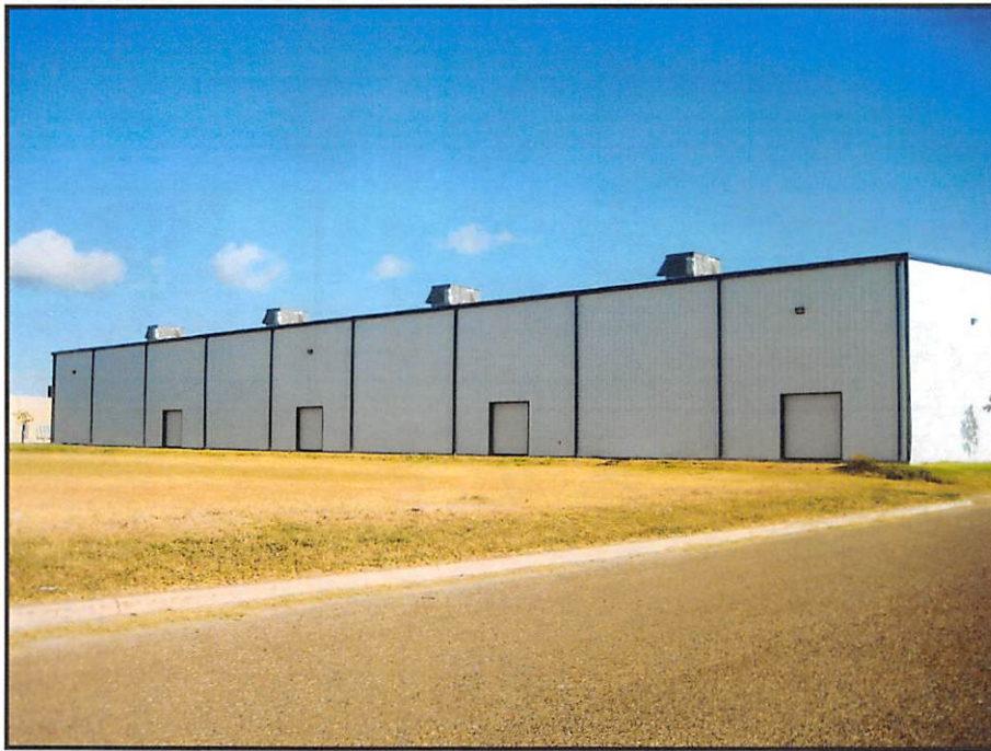
Rear View of Subject from Birch Street
