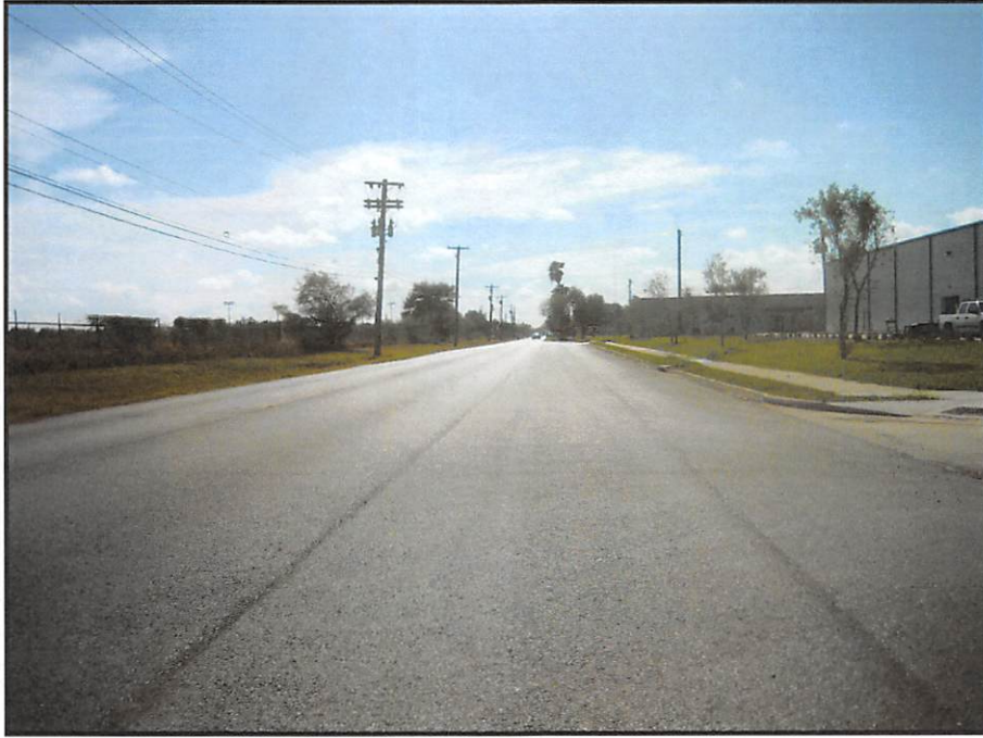
View East along Eldora Road – Subject on Right
