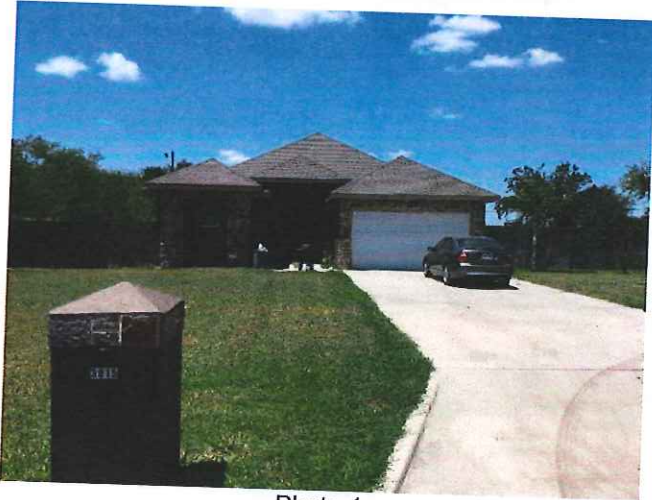
Photo 1 View of subject property
