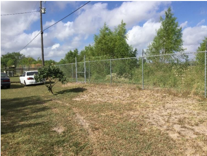
Photo 3 View of chain-link gate leading to drain ditch
