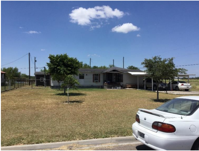
Photo 1 View of subject property
