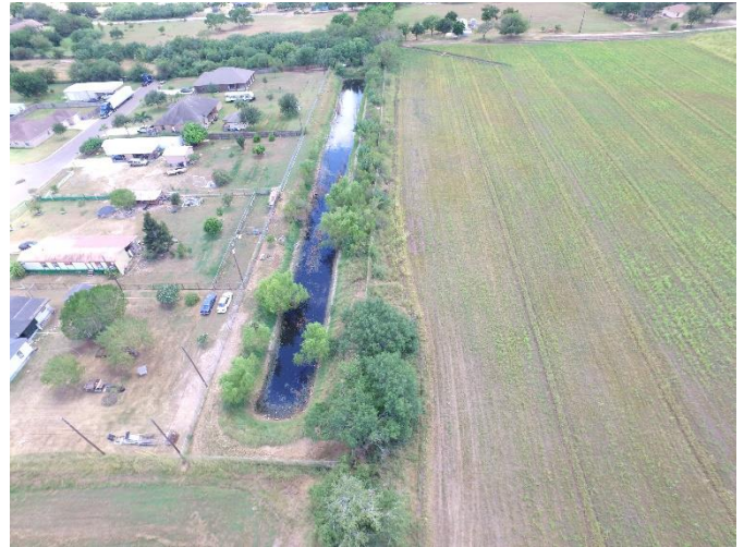
Photo 2 Aerial view of the existing detention pond by plat restriction which is also the proposed acquisition area taken by HCDD No. 1. Drone.
