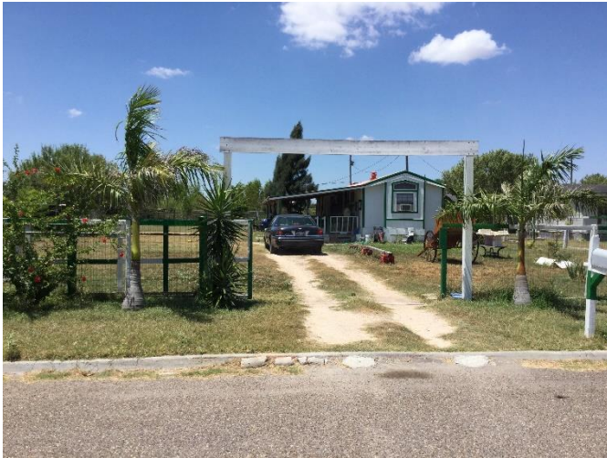
Photo 1 View of subject property
