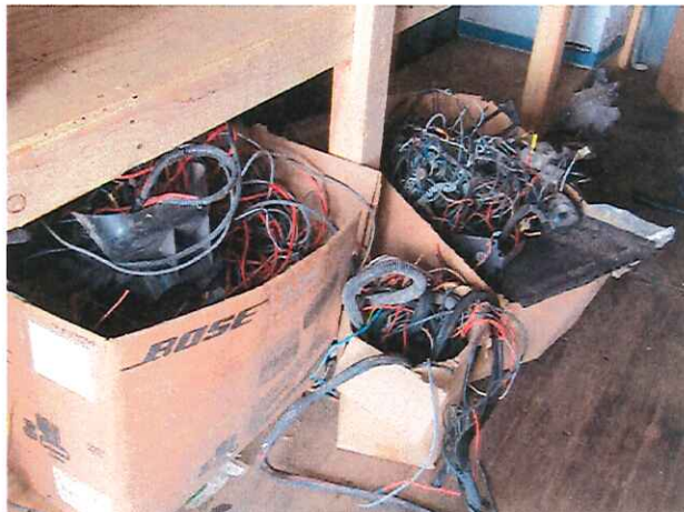
3 boxes of wires
