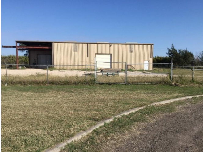
Photo 1 View of subject property
