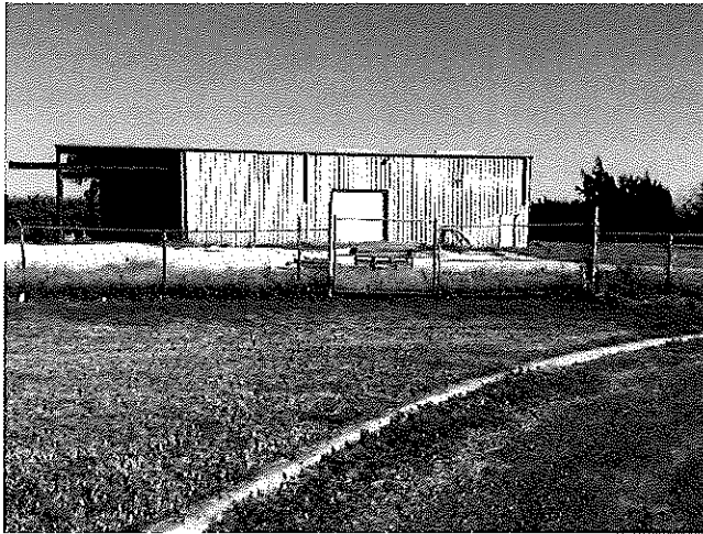
Photo 1 View of subject property
