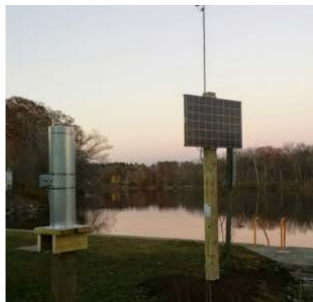
Figure A3 Standard REON RTHS station installation showing precipitation gauge, meteorological package, and solar panel
